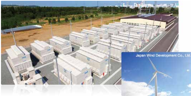
Figure 43: 34MW NaS battery operating at a 51MW wind farm in Japan 132
