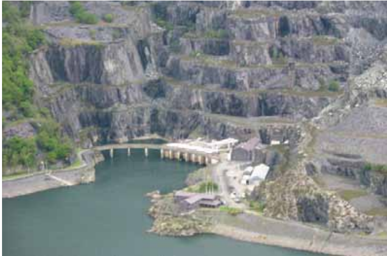
Figure 38: Outlet and inlet of the Dinorwig pumped hydro power station (and lower lake) 120
