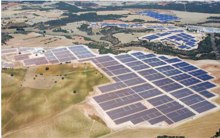
Figure 23: A large photovoltaic array in Spain
